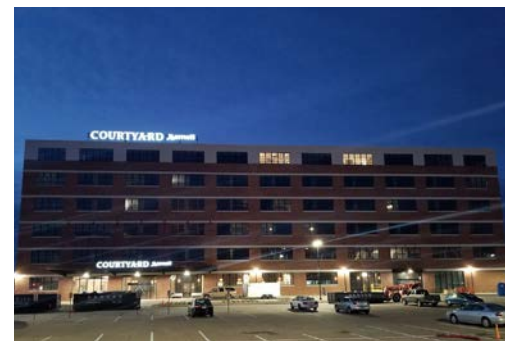
Courtyard Marriott Waterloo Cedar Falls
